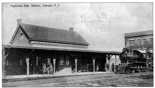
An unidentified camelback-type 4-4-2 locomotive of the DL&W eases a westbound train into Highland Avenue Station on a sunny morning around 1910. This second stop in Orange was originally called Orange Valley, but the name was changed around 1890. Built in about 1905, this station survived only about 12 years before it was demolished during the 1916–18 grade separation project. A new station was then constructed on the eastbound side.
