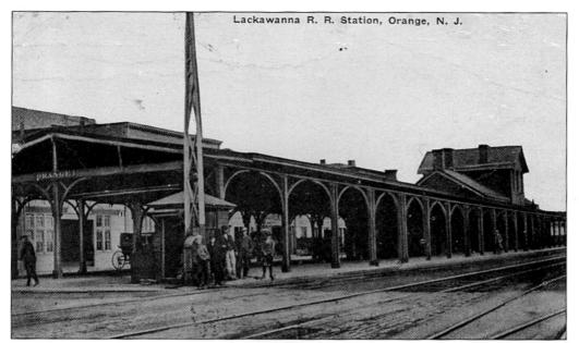
The Lackawanna Railroad rebuilt and elevated much of its line though the Oranges between 1916 and 1918 in order to eliminate grade crossings and modify curvatures and gradients. The track was realigned slightly to reduce the sharpness of the Orange Curve, necessitating demolition of this building. A new brick station was constructed just west of this site. In this view, local boys find the gateman's shanty a good place to congregate.
