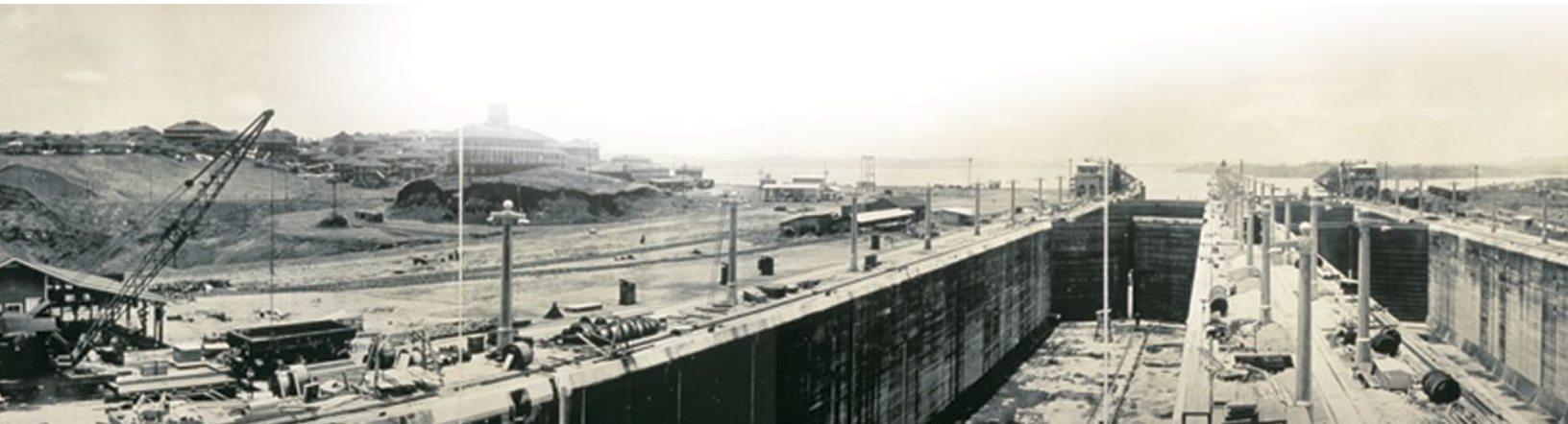
The massive Gatun Locks, shown here under construction in 1914, raise ships 85 feet onto Gatun Lake, an inland waterway on the Panama Canal.
