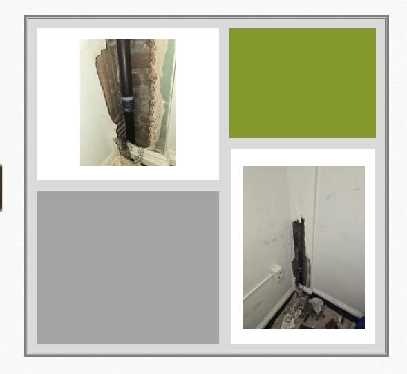
We successfully repaired a steam pipe that had ruptured within the wall.
