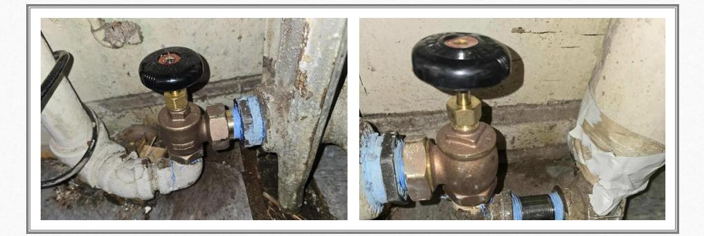
Before and after photos showing the repairs made to the steam pipes and valves.
